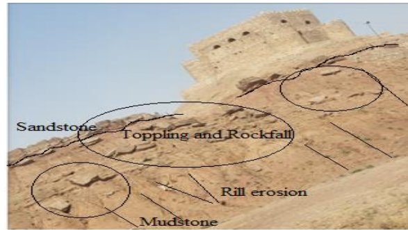
Fig. 12 Rock cliff holding on the top the historical castle of cultural heritage - Station 3 (NW view).
