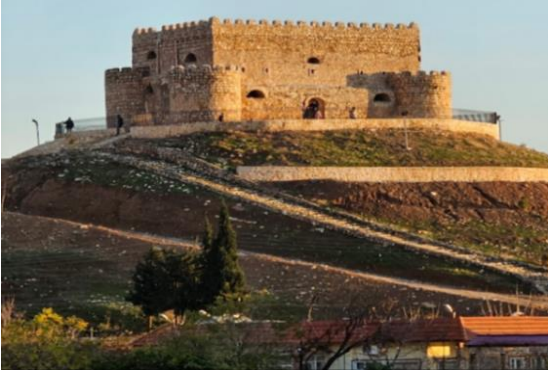
Fig. 16 The view shows a new wide road being cut, exposing the rocky slopes and the old stairway to gradual collapse.
