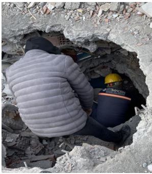
Fig. 5 Shaft-shaped search and rescue operation.
