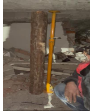
Fig. 6 Collapse control work by the use steel and wooden supports
