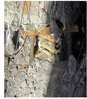
Fig. 8 Wood crib reinforced supporting work.
